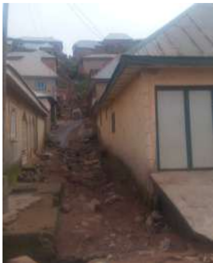
Figure 5: Undefined Drainage Path Source: Field Work, 2017
